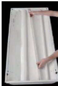
b) Remove tube lamps
